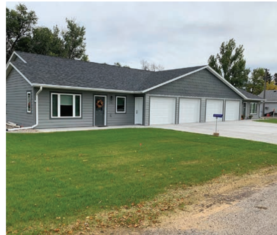
Pictured is a slab on grade stick-built twin home built in 2022. These units have three bedrooms, two baths and double attached garages with everything built for handicapped access. Two dilapidated homes on two adjacent lots were torn down by HAHD to allow for construction of these new units.
