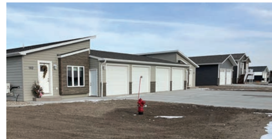
HAHD built these Dakota plex units in 2024 to create a twin home. They are three-bedroom, two-bath units purchased from South Dakota Housing Development Authority with two-stall attached garages. The 2023 Governor's House project is pictured in the background beside the twin home. HAHD currently has 16 rental units with 100% occupancy and a waiting list.
